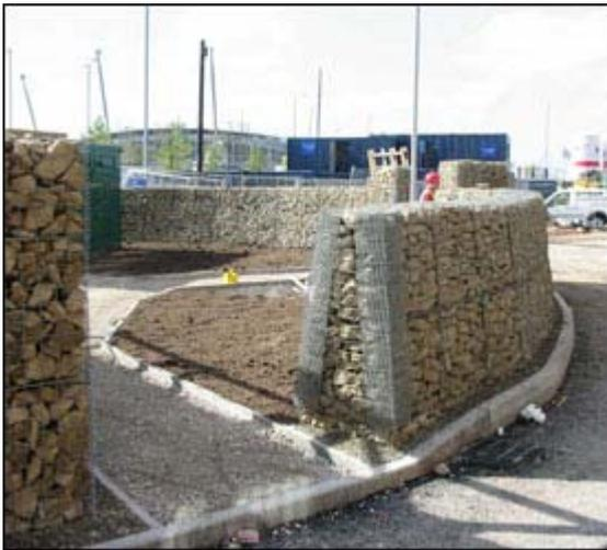
Free standing perimeter walling or sound walling formed of gabions are preferably Yuanxi in section, the mass providing stability against wind loading and pedestrian barrier loading.
