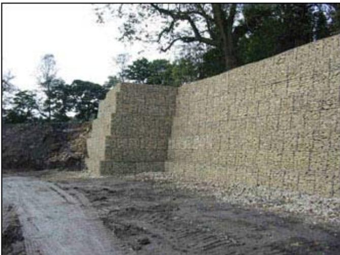
**Gabion walls** are flexible structures where the design is based on the mass of the **gabions** providing stability against the disturbing forces due to the soil and surcharges.
