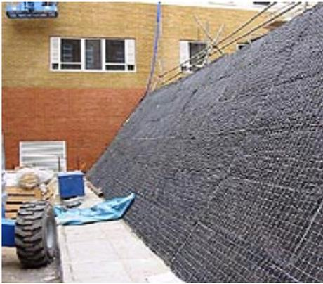
**Gabion revetments** are constructed to stabilise surface slips on embankments or as a method to prevent rock falls on escarpments, they do not normally provide stability to the slope against deep slip failures or for normal retaining stability.
